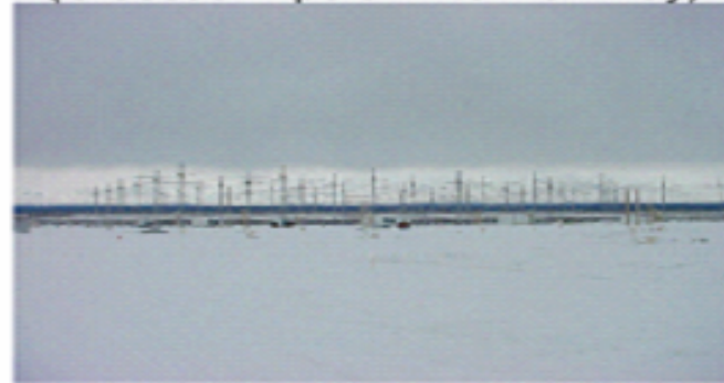
HAARP HF Transmitter (Crossed-Dipole Antenna Array)
