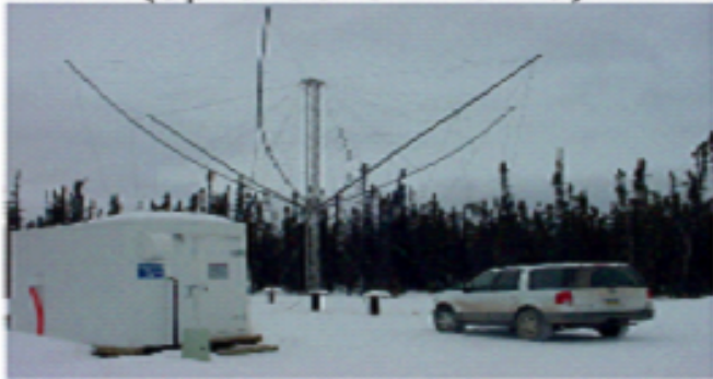
HF Receiving Station (Spira-Cone Antenna)
